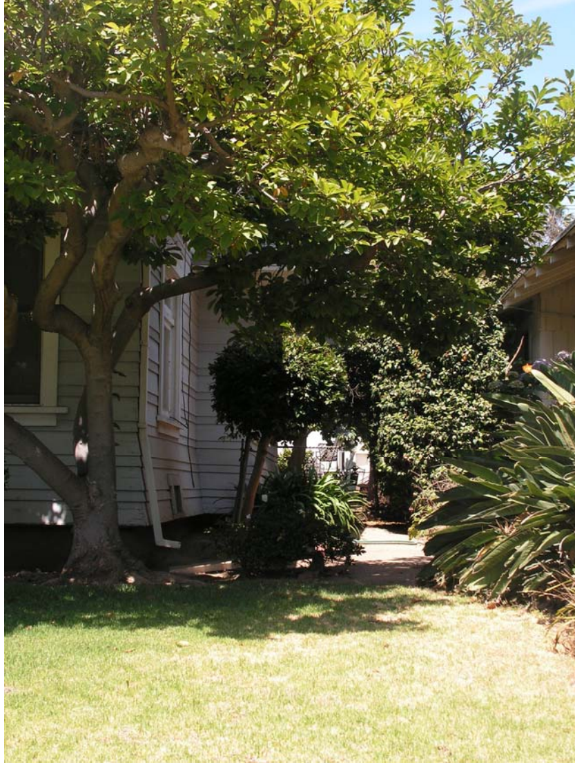
South Elevation, View Northeast.
