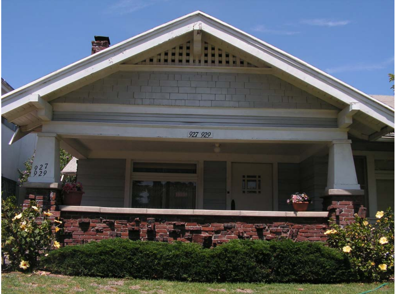
Front (West) Elevation, View East.
