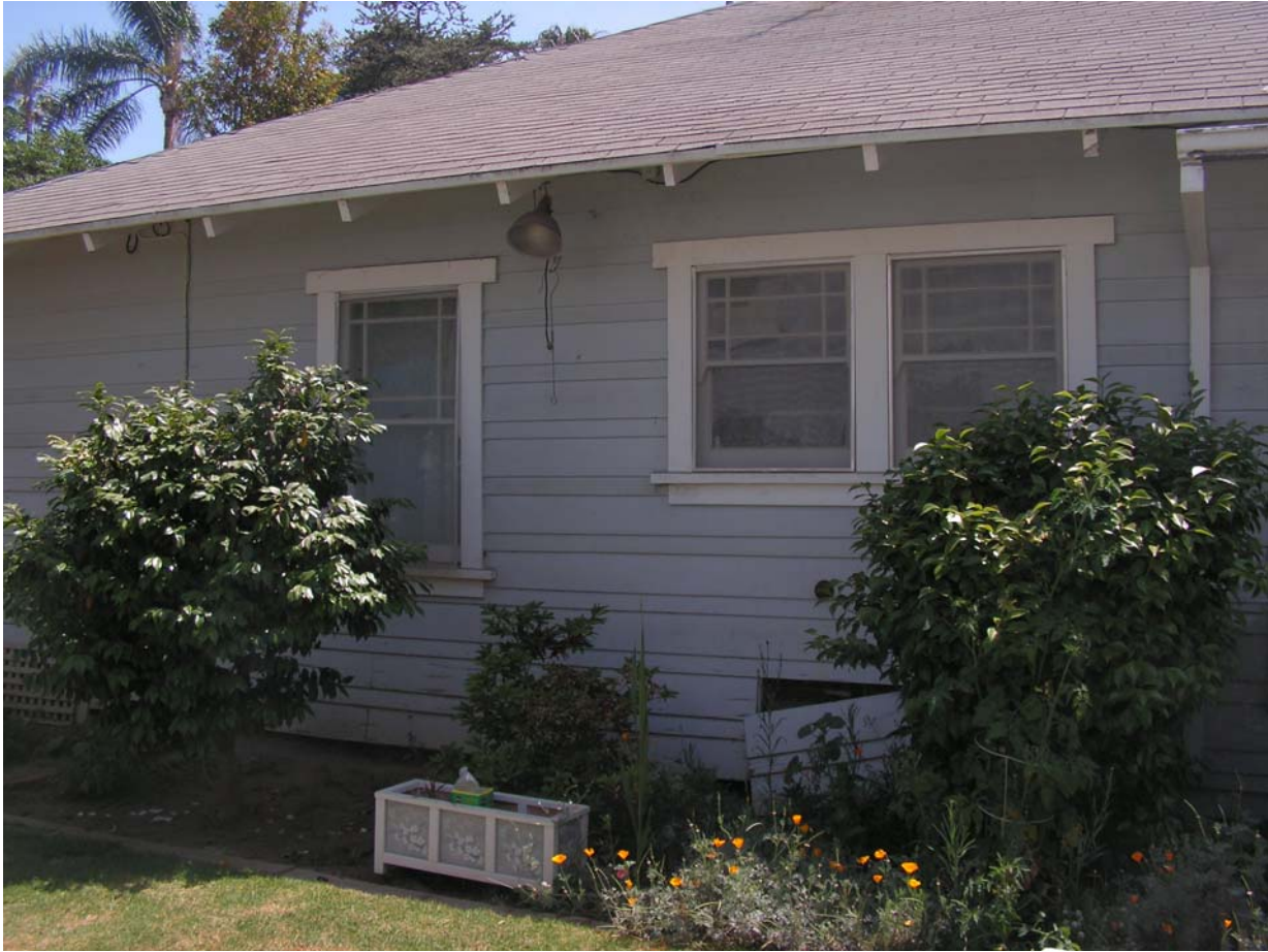
East Elevation, View Southwest
