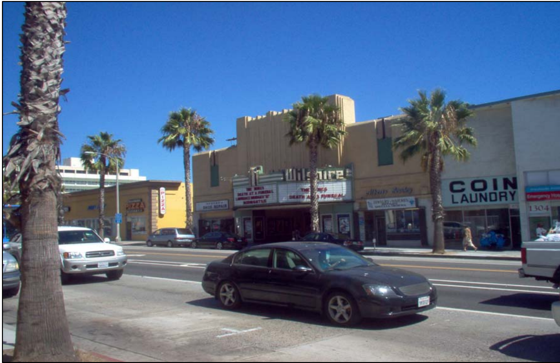
Perspective view showing the primary (north) elevation, view southeast.
