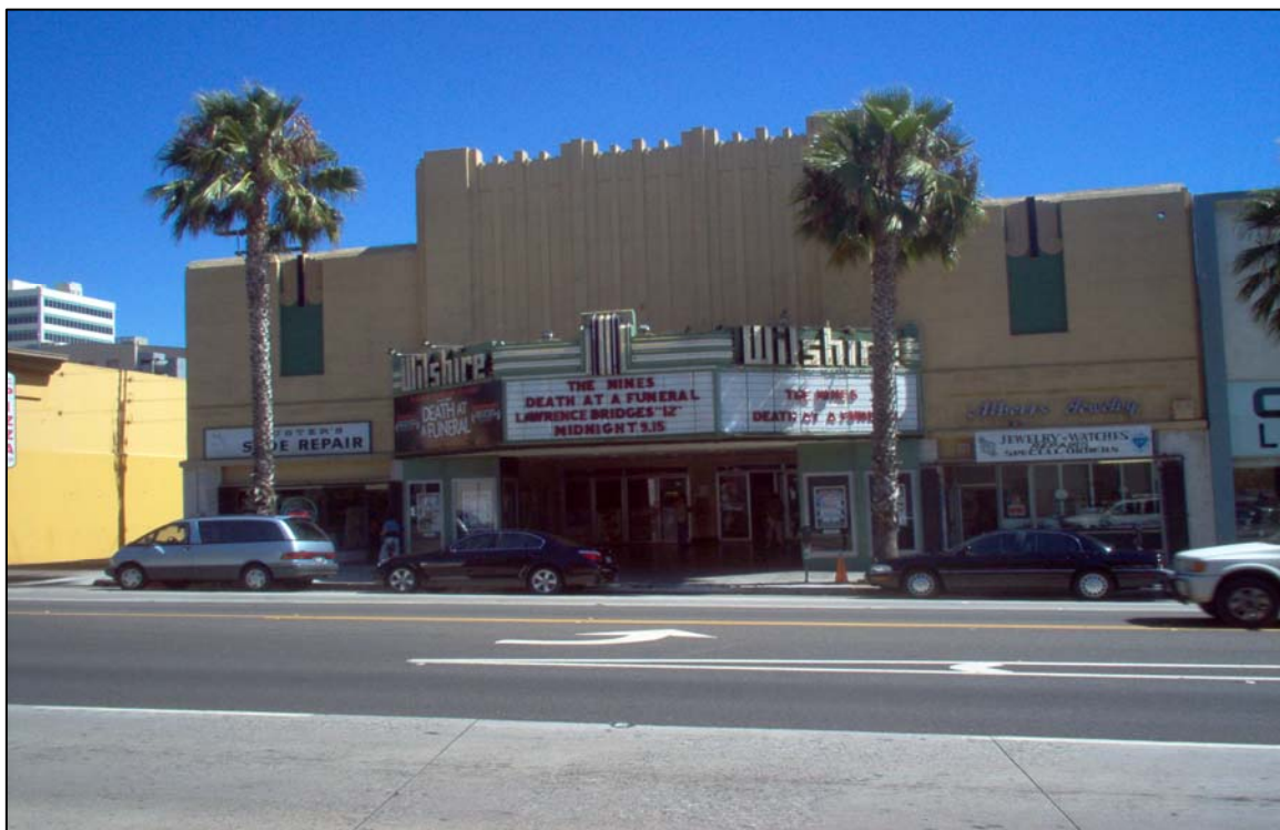
Primary (north) elevation, view south.
