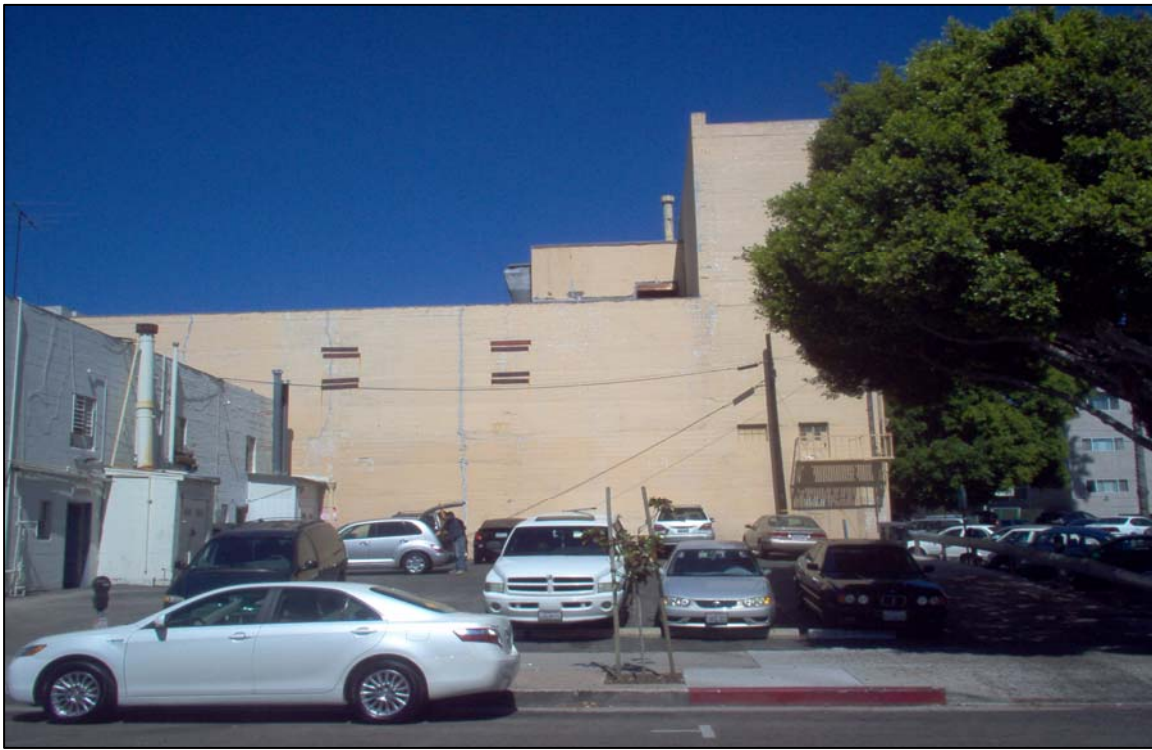
West side elevation, view east.
