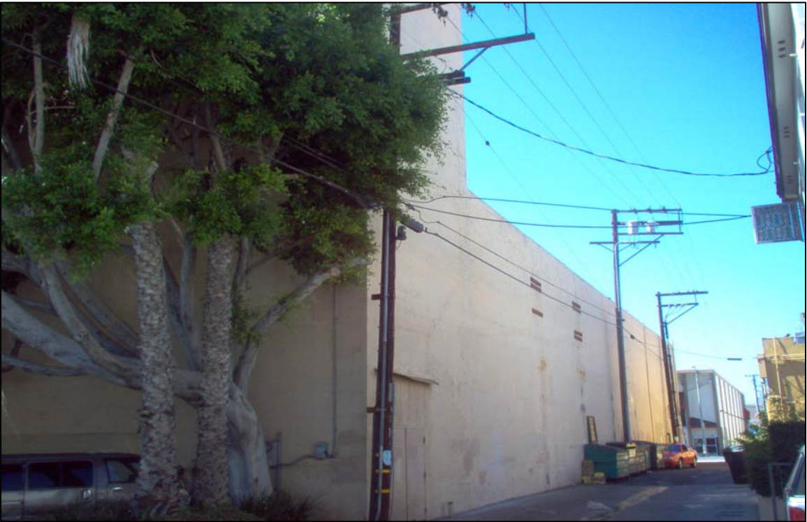
East side elevation, view north.
