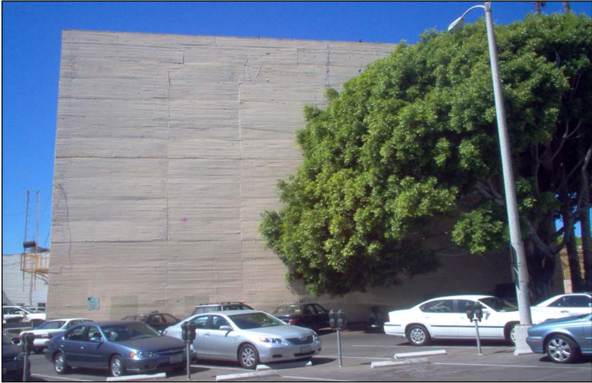
Rear (south) elevation, view north.
