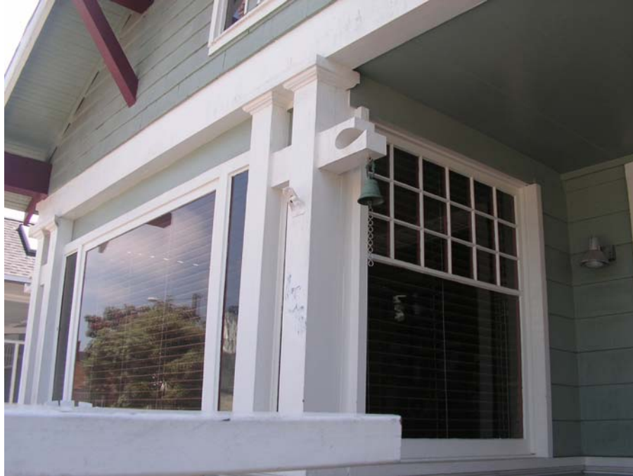
Enclosed porch, looking southeast
