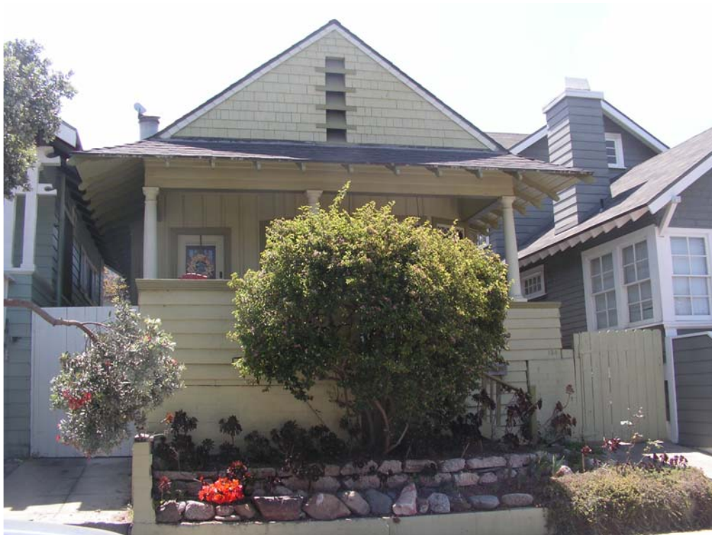
Primary (north) façade 134 Hart Avenue, looking south
