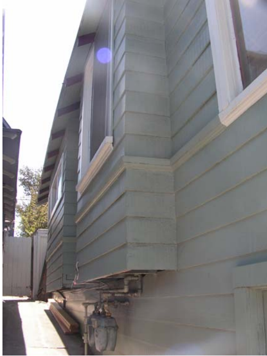
Secondary (east) elevation, looking southwest
