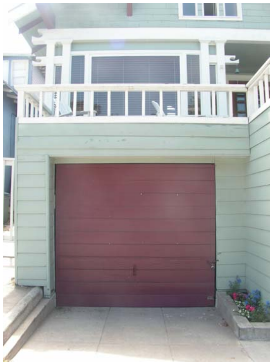
Garage, looking south
