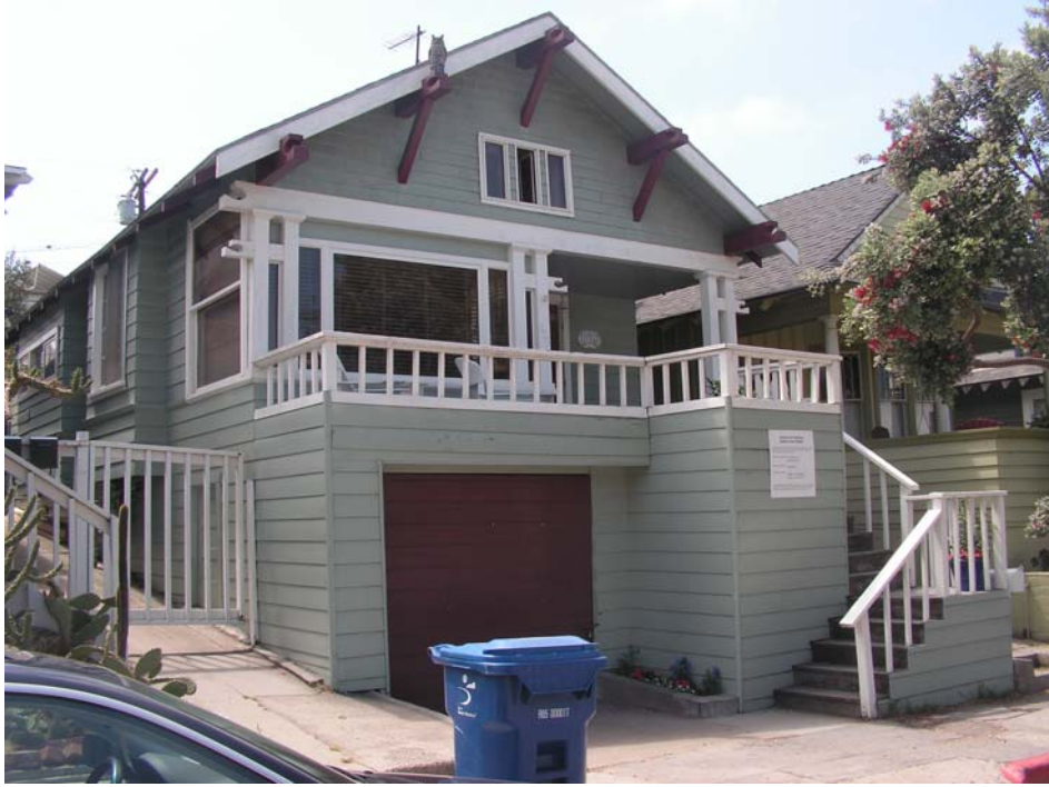
Primary (north) elevation, looking south
