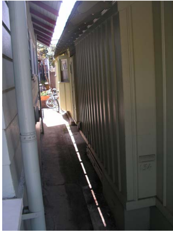
Secondary (west) elevation, looking south
