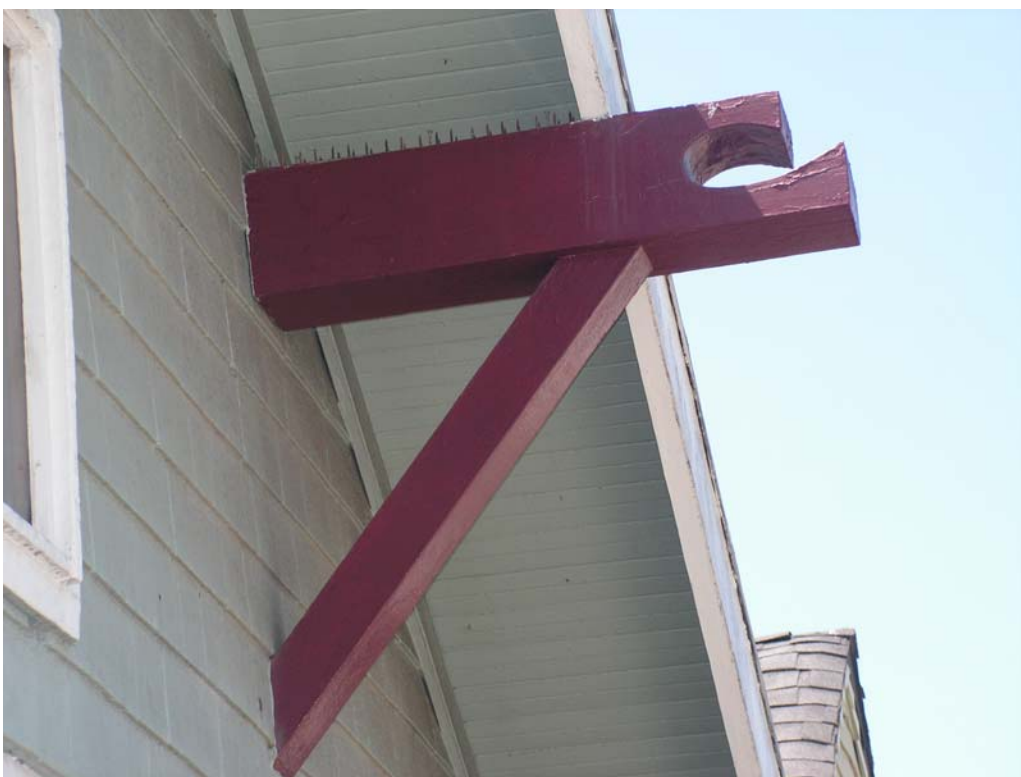
Bracket, looking southwest
