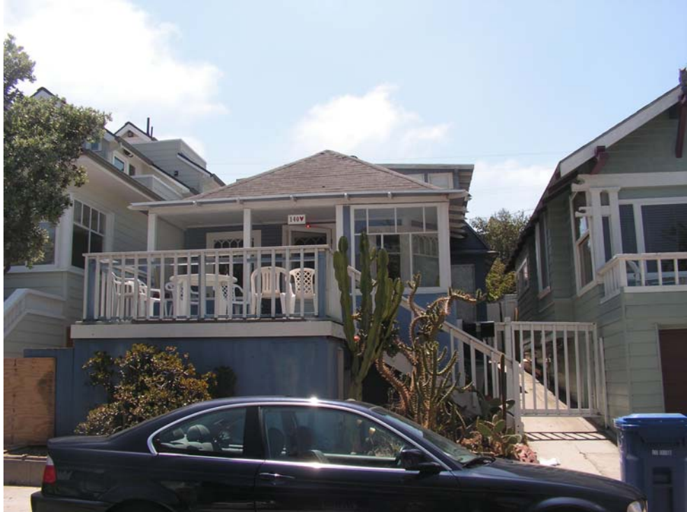
Primary (north) façade 140 Hart Avenue, looking south
