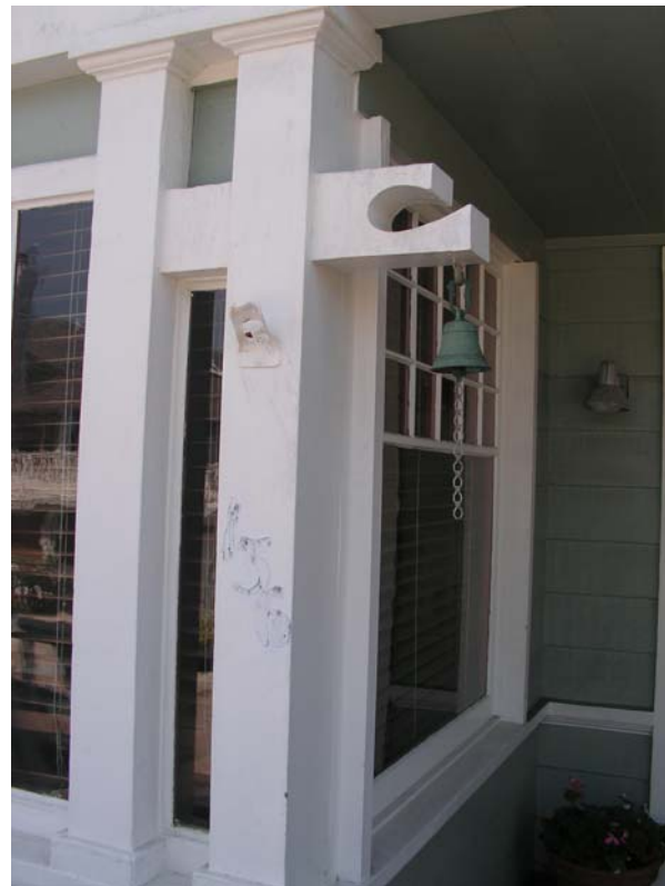
Box-posts, looking southeast
